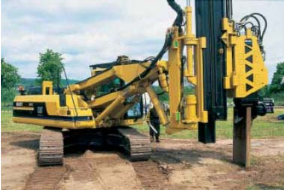
Sheet-wall piling equipment
