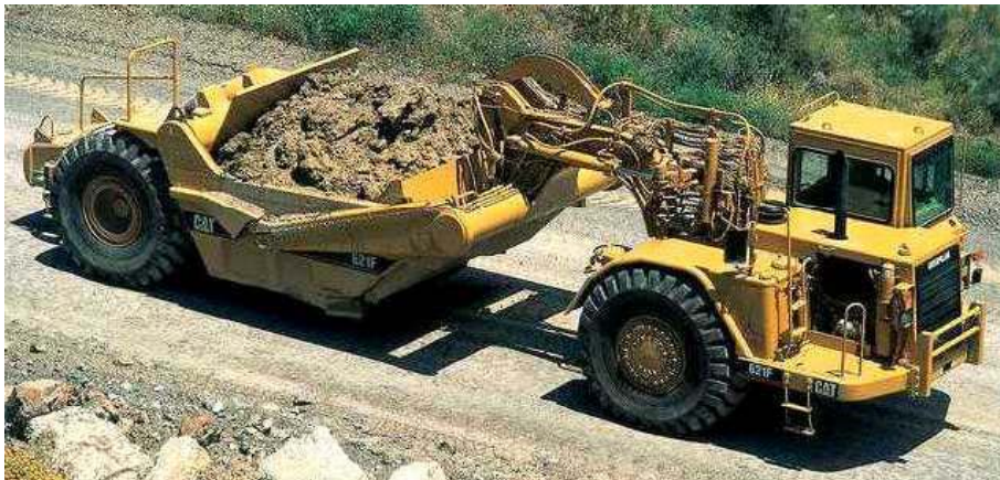
Hauling excavated soil
